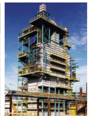
Ethylene Cracker Unit
