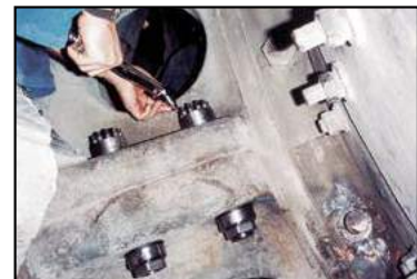
Split gear segment on rotary kiln.
