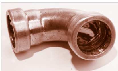
FIGURE 63: Permanent push-connect fitting
